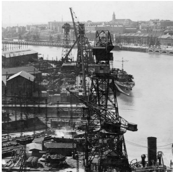
Chantiers navals Dubigeon
